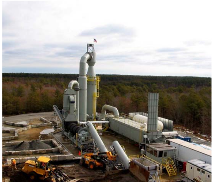
Thermal desorption unit at Demolition Area 1
