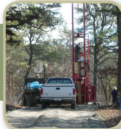
Monitoring well drilling
