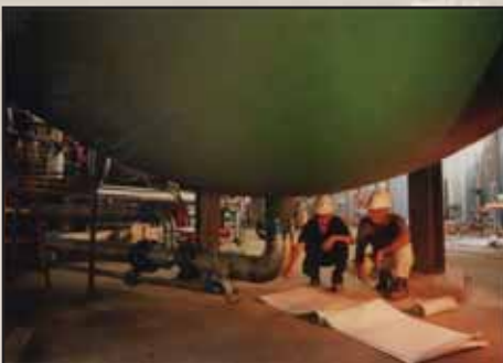
Inspection of granular activated carbon treatment vessel.
