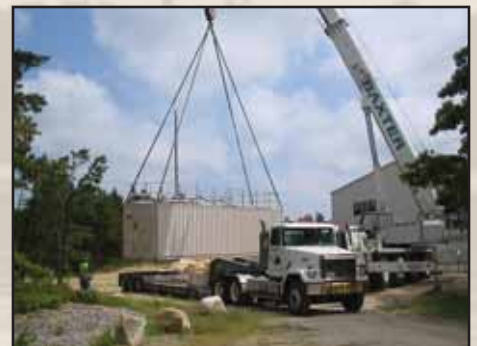
A modular treatment unit is moved for reuse at another plume site.
