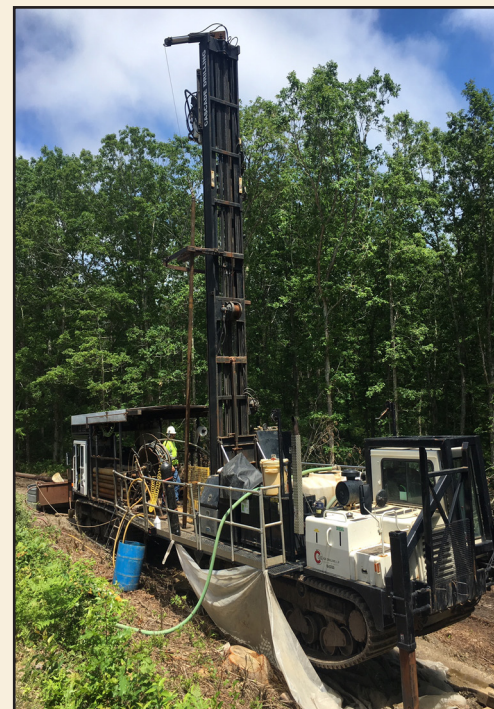
A sonic drill rig collects groundwater samples up to 300 feet deep.
