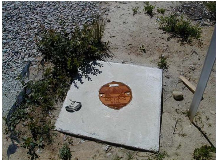
Photo of a finished well site
