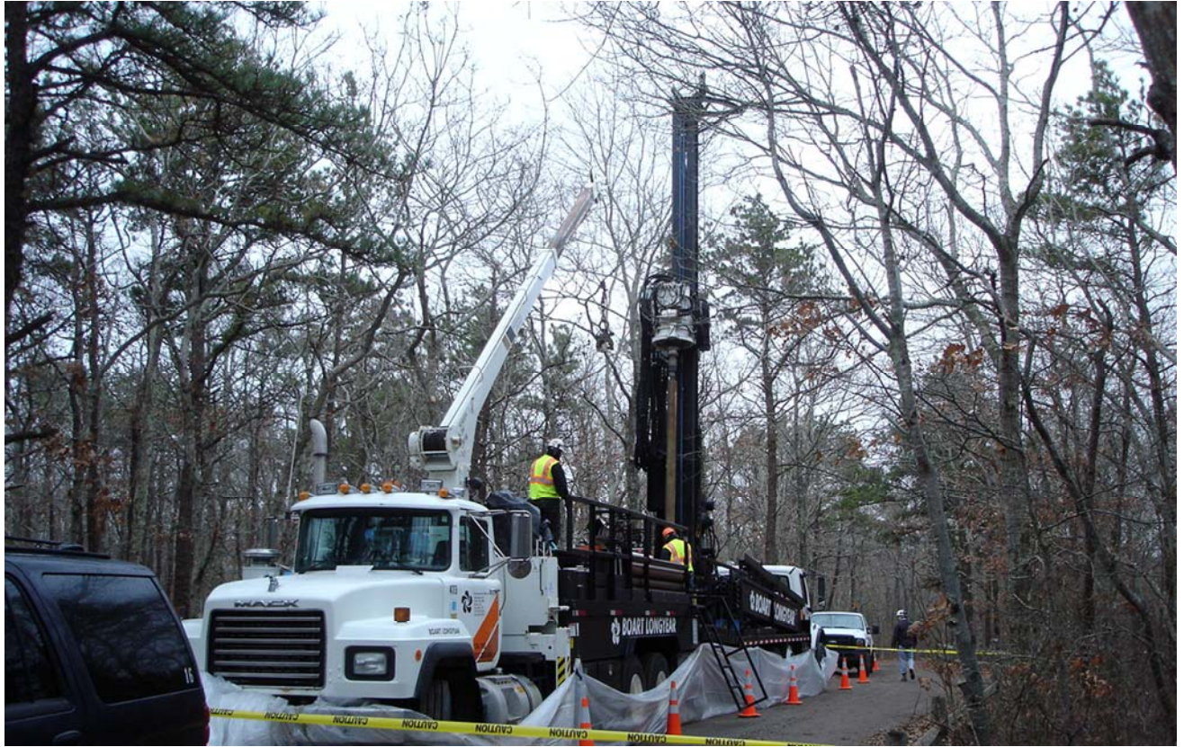
Photograph of drill rig and equipment
