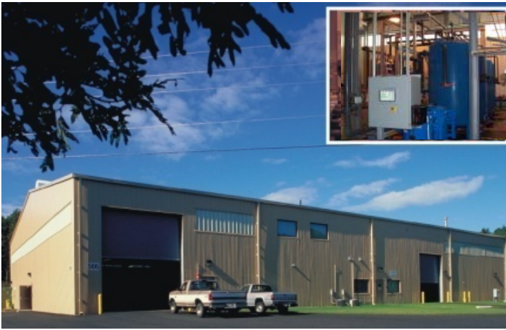
J-3 Groundwater Treatment System is Housed in AFCEC's FS-12 Facility
