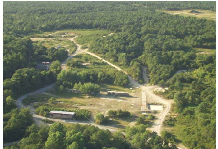
J-3 Range Prior to the Demolition of Structures
