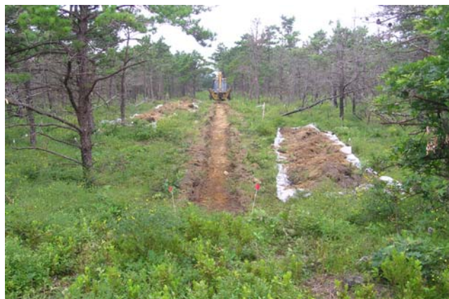
Former K Range - Trench
